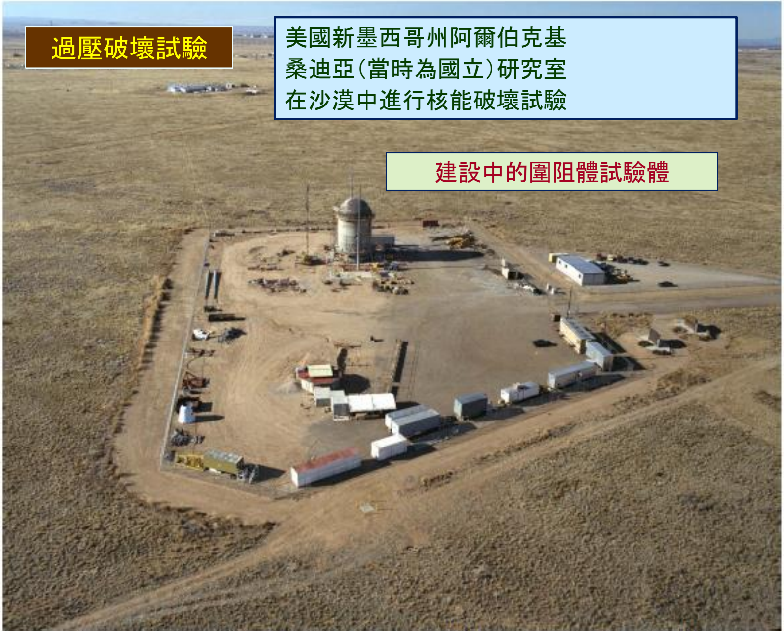
Figure 2.11 Aerial View of CTTF-West during PCCV Construction (March, 1999)
