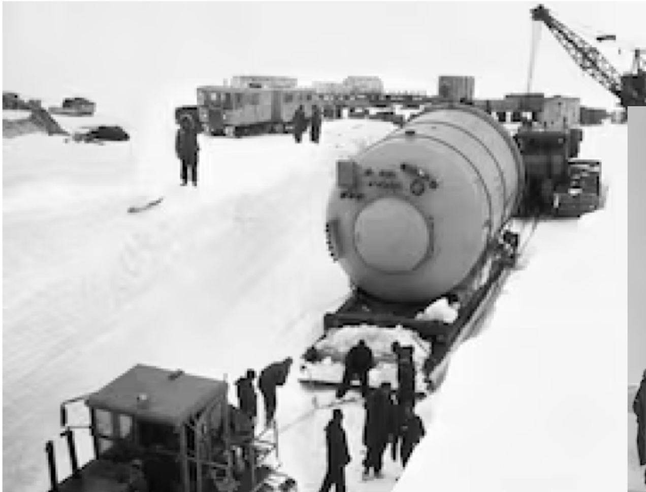
U.S. Army Engineers install move a vapor condenser, part of a portable nuclear power plant. Bettmann Archive/Getty Images
